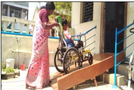
Ramp at the entrance
